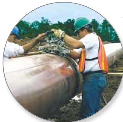
*The PipeWIZARD® is specifically designed for the automated inspection of pipeline girth welds using phased arrays for fast weld-to-weld inspection.*
